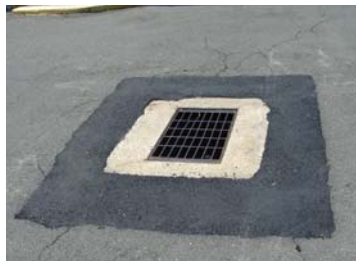
Catch Basin Top Repair
