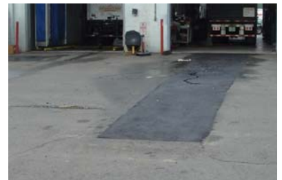
Trench Cut Repair
