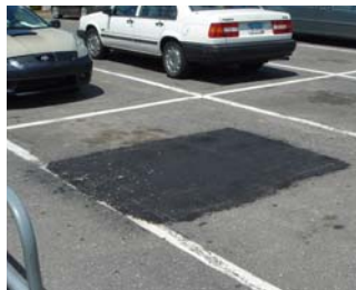
Pot Hole Repair
